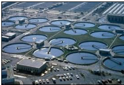
An aerial (from above) view of a sewage treatment plant.
